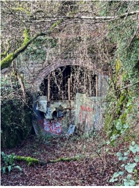
If you take a few minutes to continue along this track you can see the original tunnel, now mostly boarded up.
